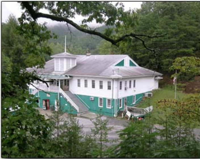
Sunset Gap Community Center
